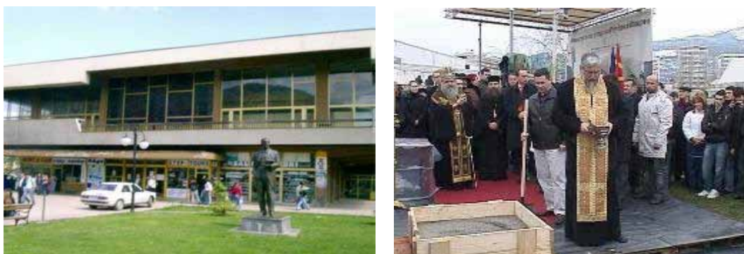
Photo 2. The Cultural Center (Tetovë) build on the spot of the old mosque and the foundation stone of Philharmony on the spot of Ibn Pajko mosque
