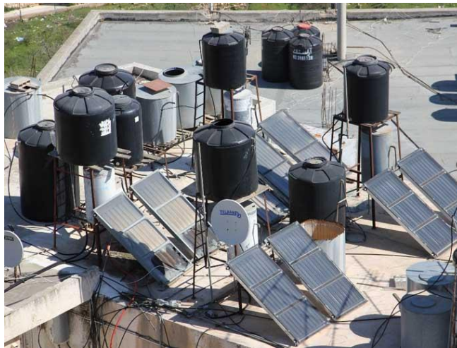
Figure 1.25: A Palestinian building's roof showing water tanks (Url-12).
