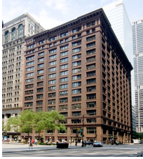
Şekil 25 Holabird and Roche: Marquette Building. Chicago. 1893 – 94.
