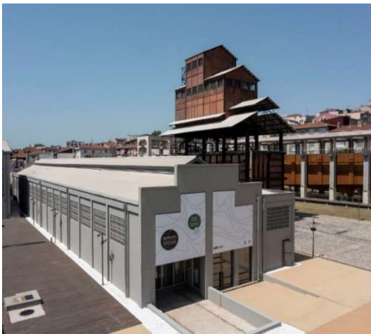
Figure 2. 24: Exhibition space, block P, refunctioned original structure (URL-25).
