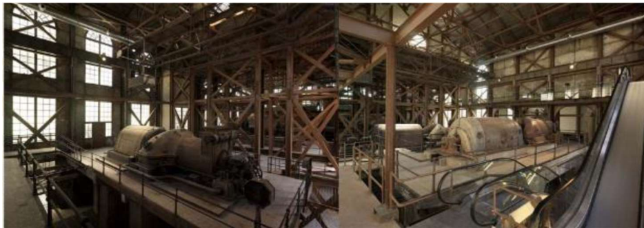
Figure 2. 11: The steel framework and the original machines with minimum interventions (URL-20)
