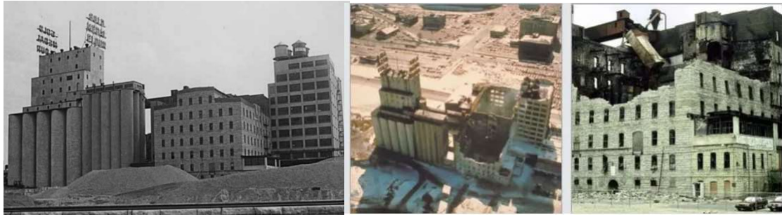
Figure 2. 3: Abandoned Washburn A Mill (URL-18), 1976, day after the fire 1991, ruin 2000 (URL-34).
