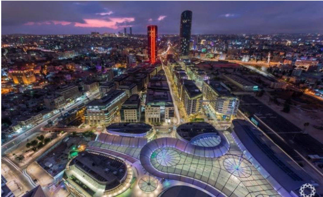
Figure 10 Al-Abdali Boulevard Project, Amman (Al-Abdali Group Procure, 2019)
