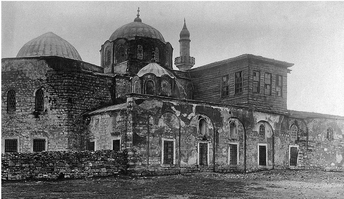
Fig. 9 Fethiye Camii, North Façade, Sender, 1925 (DAI, neg. no. 31897).
