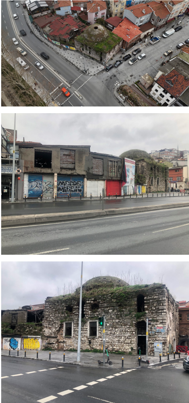
Fig. 3. (a) Aerial photograph; (b-c) coastal road facade of the Ayakapı Bath (Photos: Authors, 2025)
