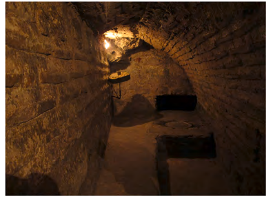
Fig. 19 Muhliotissa, Kimiseos tis Theotokou hagiaσμα, recessed brick technique (Esmer, 2017).
