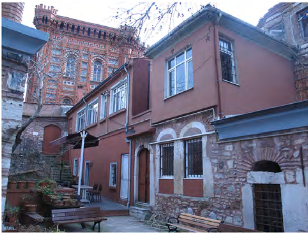
Fig. 14 Muhliotissa, annex building (Esmer, 2017).
