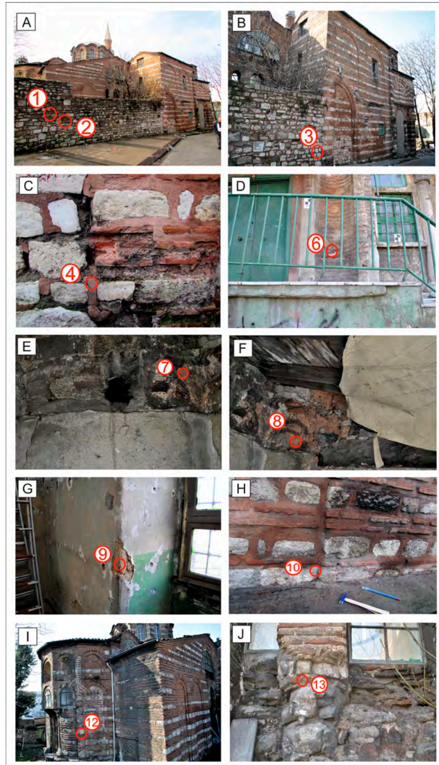
Figure 3. Sampling locations of the mortar samples. (A) Outer face of the northern garden wall (MG-1 and MG-2). (B) Lower level of the corner wall of the northern annex (MG-3). (C) Lower level of the semi-arched niche on the northern annex façade (MG-4). (D) Lower level of the niche to the right of the main entrance door on the entrance façade (MG-6). (E) Upper level of the oval minaret base inside the tomb structure on the southern façade (MG-7). (F) Upper level of the wall to the right of the minaret base on the southern façade (MG-8). (G) Interior wall surface of the entrance portico on the west side (MG-9). (H) Lower level of the exterior façade at the southeastern corner (MG-10). (I) Exterior face of the qibla wall (eastern façade, apse) (MG-12). (J) Between the brick and stone elements on the northern exterior façade (MG-13).
