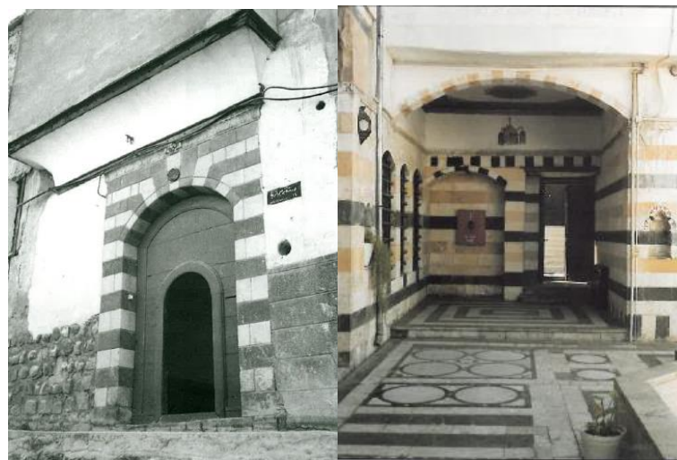
Figure 3.2: On the left door's photo of Zain Al-Abideen House and on the right the Entry of Nizam House (Kibrit, 2000).
