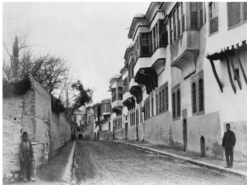
Figure 4.29: Salihyya houses with cantilevers and Mashrabiya in the upper part (Agoston & Masters, 2009).
