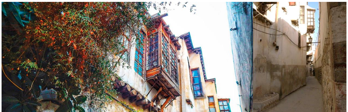
Figure 4.12: Damascene house windows from the outside. (Url-10).
