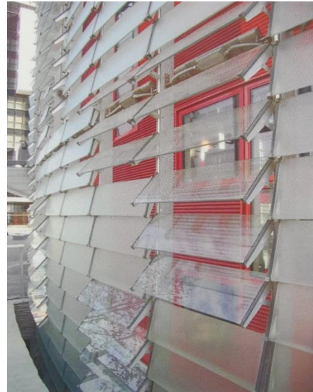
Image 2.14: Torre Agbar Tower's Double-Skin Facade Louvers (Eren, 2019).
