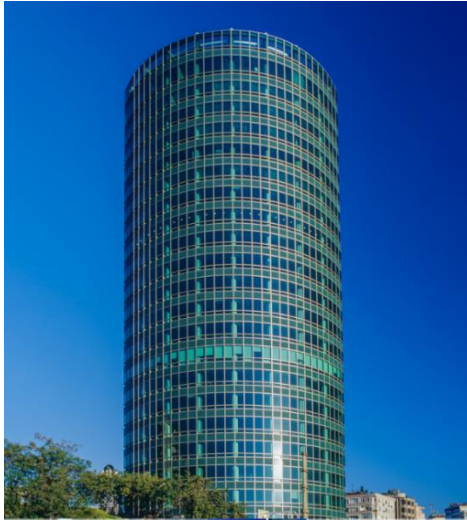
Image 3.45: Olive Grove Tower's Curtain Glass Facade System – Southern Facade, (Metal Yapı, Url-68).
