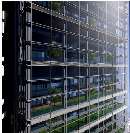
Image 2.32: Istanbul Sapphire Tower, Facade Natural Ventilation Grill (Url-22).
