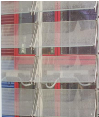
Image 2.15: Torre Agbar Tower's Double-Skin Facade Shutters Detail (Eren, 2019).
