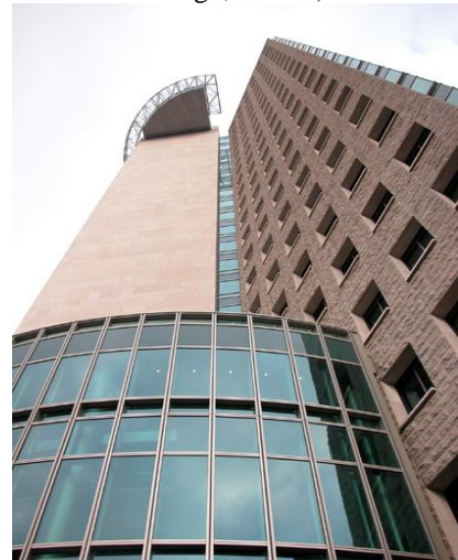
Image 3.48: Olive Grove Tower's Curtain Glass Facade System – Western Facade (GKV Architects, Url-53).
