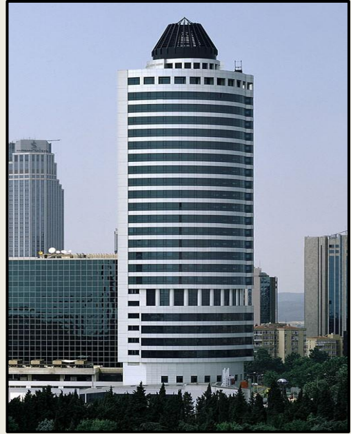
Image 3.40: Metrocity Office Tower (Url-66).
