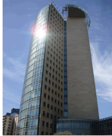
Image 3.46: Olive Grove Tower's Curtain Glass Facade System – Eastern Facade, (Antre Design, Url-69).
