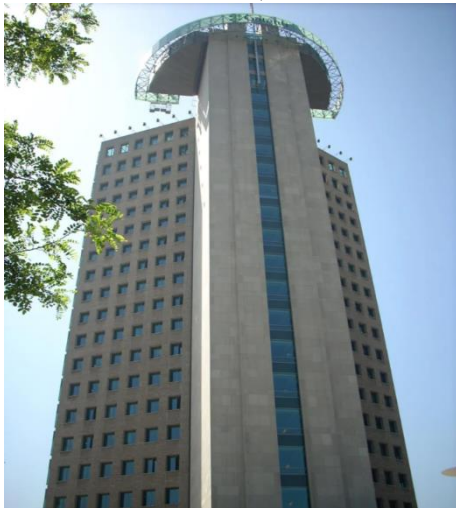
Image 3.47: Olive Grove Tower's Curtain Glass Facade System – Northern Facade (Architizer, Url-70).
