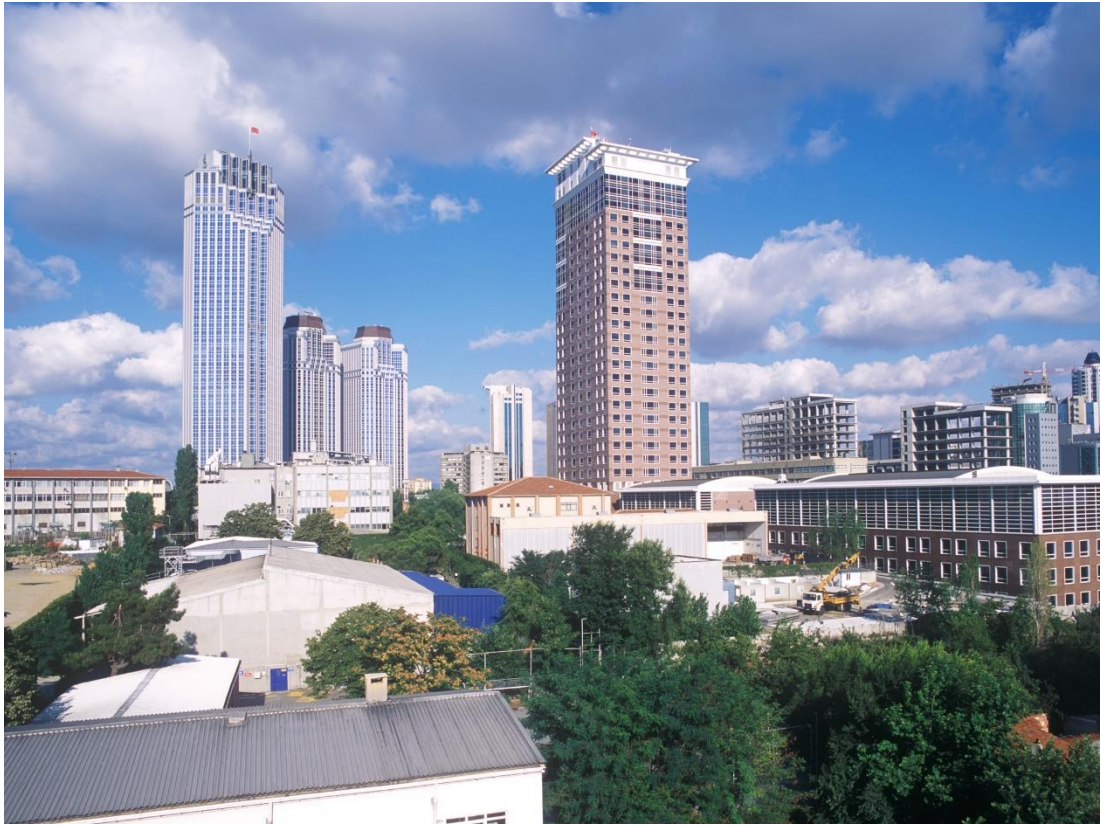
Image 3.33: Tekfen Tower's Northern and Western Facades (Url-64).
