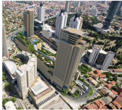
Image 3.64: River Plaza, Northern Facade (Url-49).
