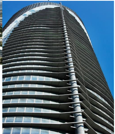
Image 3.57: Spine Tower, Western Facade, Horizontal Sunshade Elements (Url-73).
