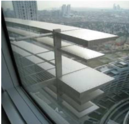
Image 3.28: Kanyon's Facade Shading Element From The Inside (Schulze, 2015).
