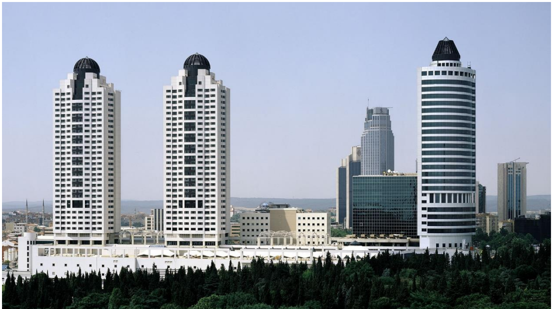
Image 3.42: Metrocity Office Tower (Url-67).
