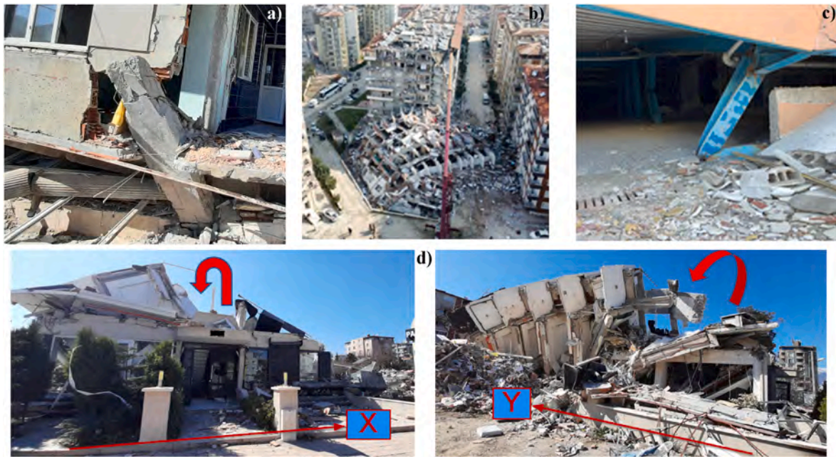
Fig. 30. Views of damaged/collapsed buildings illustrating the vertical seismic effects [13].
