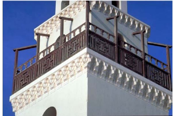
Image 2.46: The parapet on the minaret by Mohammad Akram. Source (Aga Khan Award for Architecture: Url-22).
