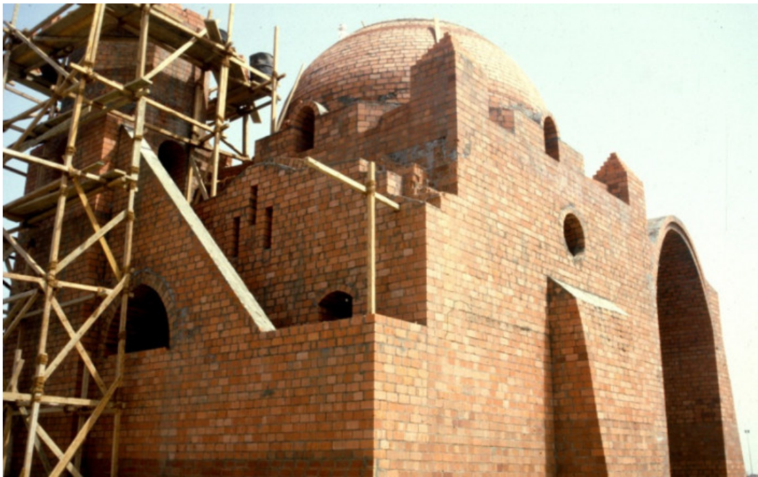
Image 2.112: Construction of the Corniche Mosque (Url-45).
