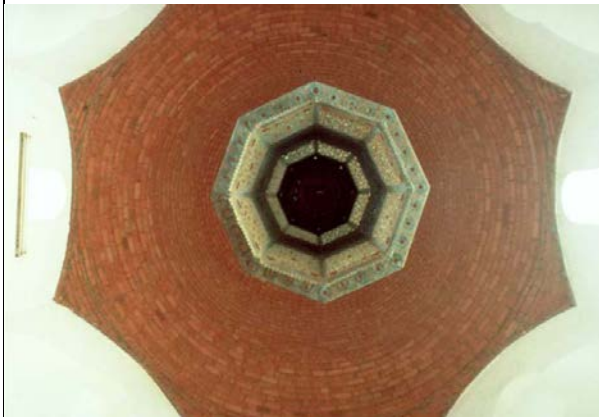
Image 2.84: Corniche Mosque Dome (The Aga Khan Award for Architecture, 1989).
