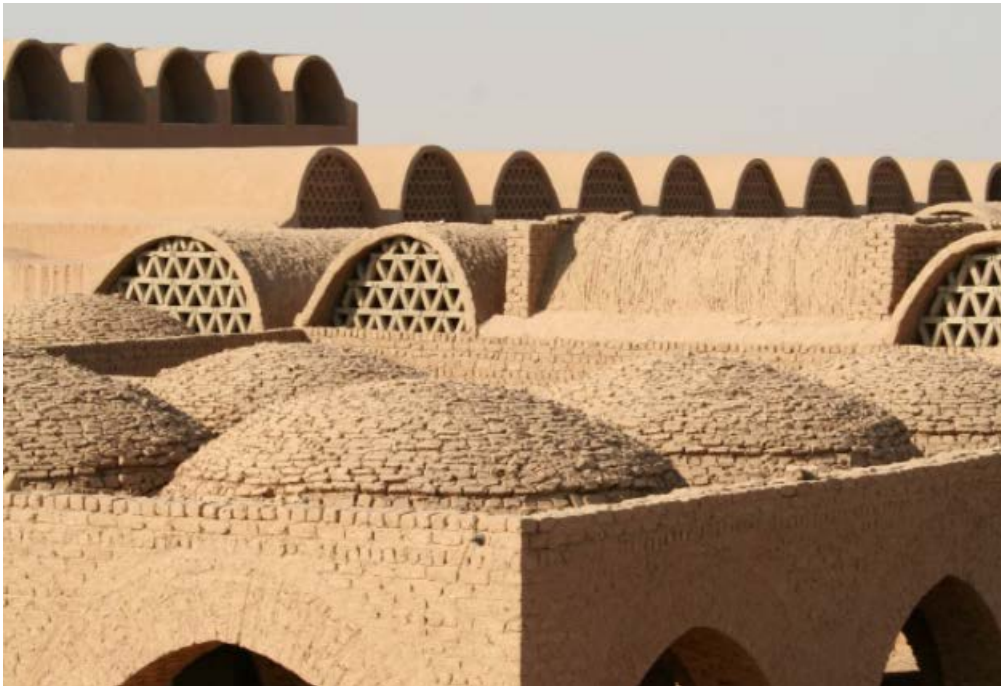
Image 2.120: Souk, New Bariz, Egypt, 1967, air inlets. Source: (Url-30).
