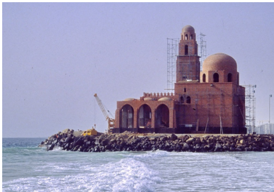
Image 2.69: Island mosque: Construction (Url-25).
