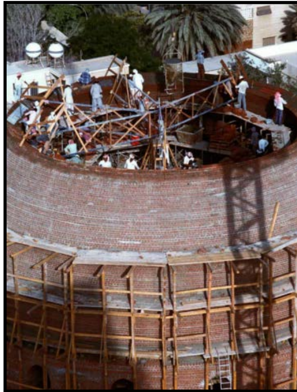
Image 2.27: King Saud Mosque: During construction (Amjad nahid, 2009).
