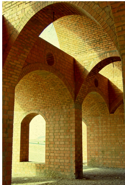
Image 2.127: Ruweis Mosque: vaults during construction (Url-32).
