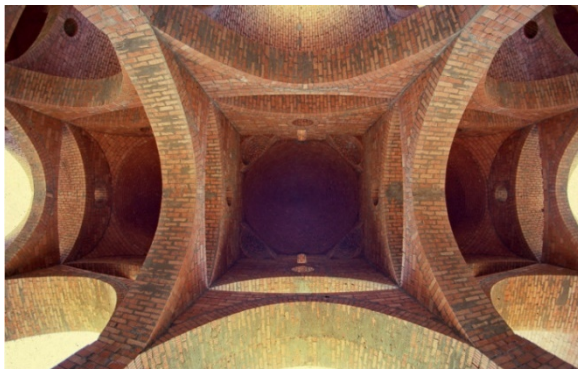
Image 2.132: Ruwais Mosque during construction (Url-32).
