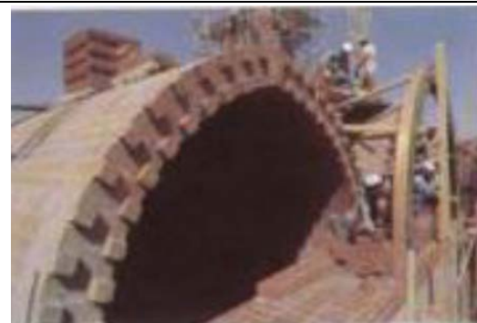
Image 3.6: Qiblatain Mosque, dome construction. Source (Aba Alkhil, 1987).
