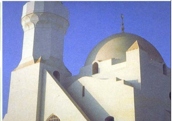
Image 2.85: Detail, stairs leading to the minaret, by Mohammad Akram (The Aga Khan Award for Architecture, 1989).
