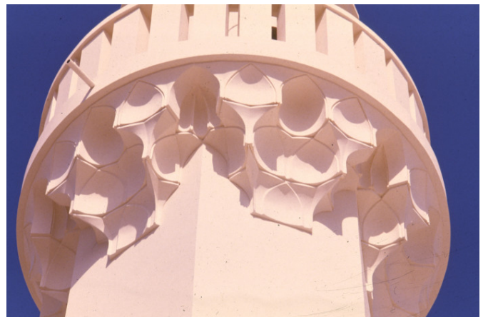
Image 2.166: Binladin mosque: Minaret balcony supported by muqarnas vaults. Source (Url-40).
