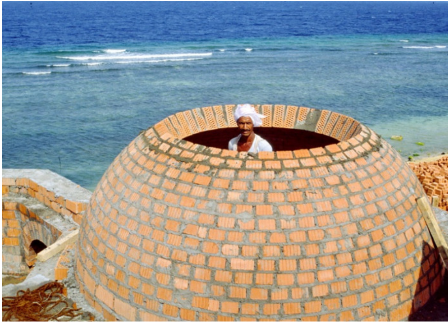
Image 2.70: Main Dome during construction (Url-25).
