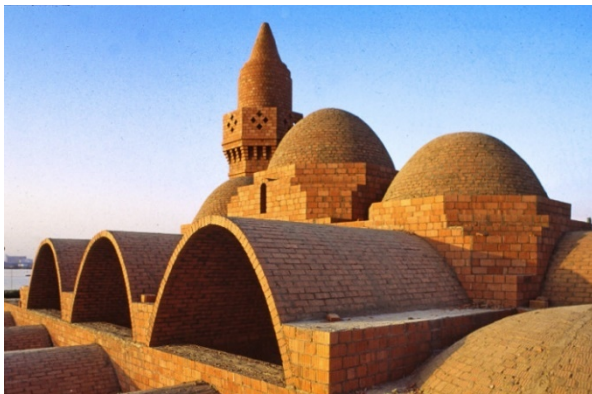
Image 2.128: Ruweis Mosque: vaults during construction (Url-32).
