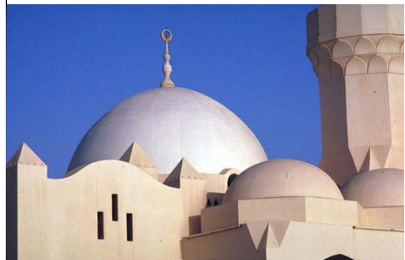
Image 2.89: Rooftop, sculptural forms, by Mohammad Akram (The Aga Khan Award for Architecture, 1989).
