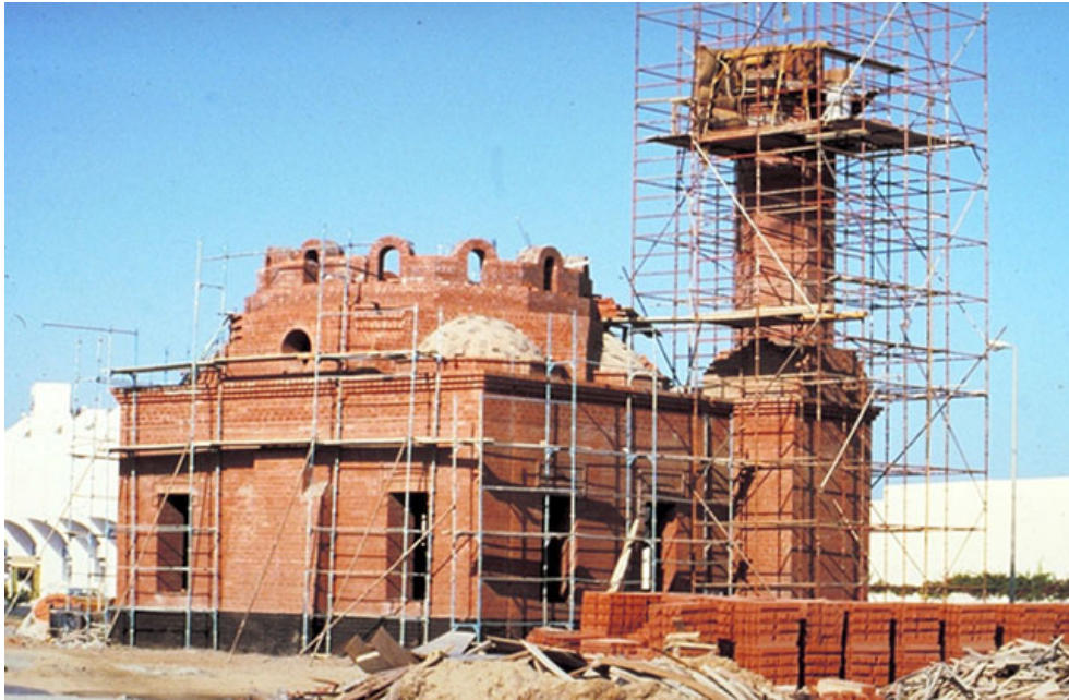
Image 2.171: Binladin mosque: Mosque during construction. Source (Aga Khan Award for Architecture, 1989).
