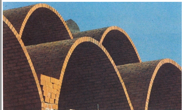
Image 2.129: Ruweis Mosque: vaults during construction (Url-32).
