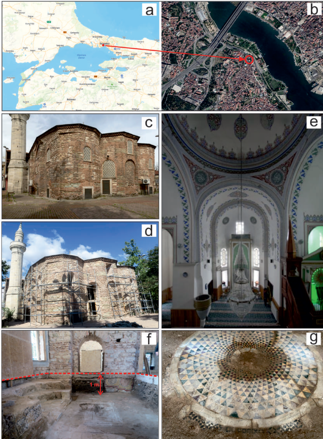
Figure 1. a) and b) 2 Map of the location of the Atik Mustafa Pasha Mosque; c) and d) Overview of the mosque before and during restoration; e) A view of the dome, mihrab, minbar, and decorative patterns inside the mosque before restoration; f) Image showing the floor level of the mosque (marked with a red line), raised more than 1 m above the original floor level of the church during the Ottoman period; g) Mosaic decoration of the original ground floor of the Byzantine church.
