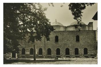
Fig. 1 The front façade of the Outer Treasury after the restoration in 1933 (Altındağ and Bayraktar, 1988). The opened understratum windows had been refilled in an unknown date.
