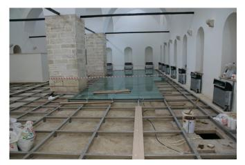
Fig. 5 Covering the original floor with glass panels.
