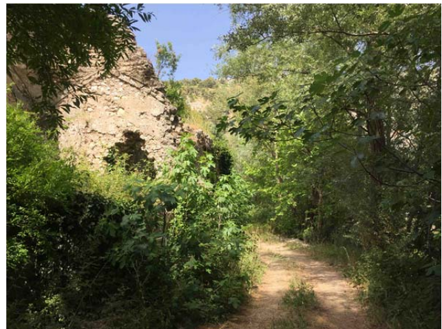
Figure 7. Hammam in Blagaj showing a lack of maintenance and the poor presentation of the national monument (Source: Sabanovic N.)
