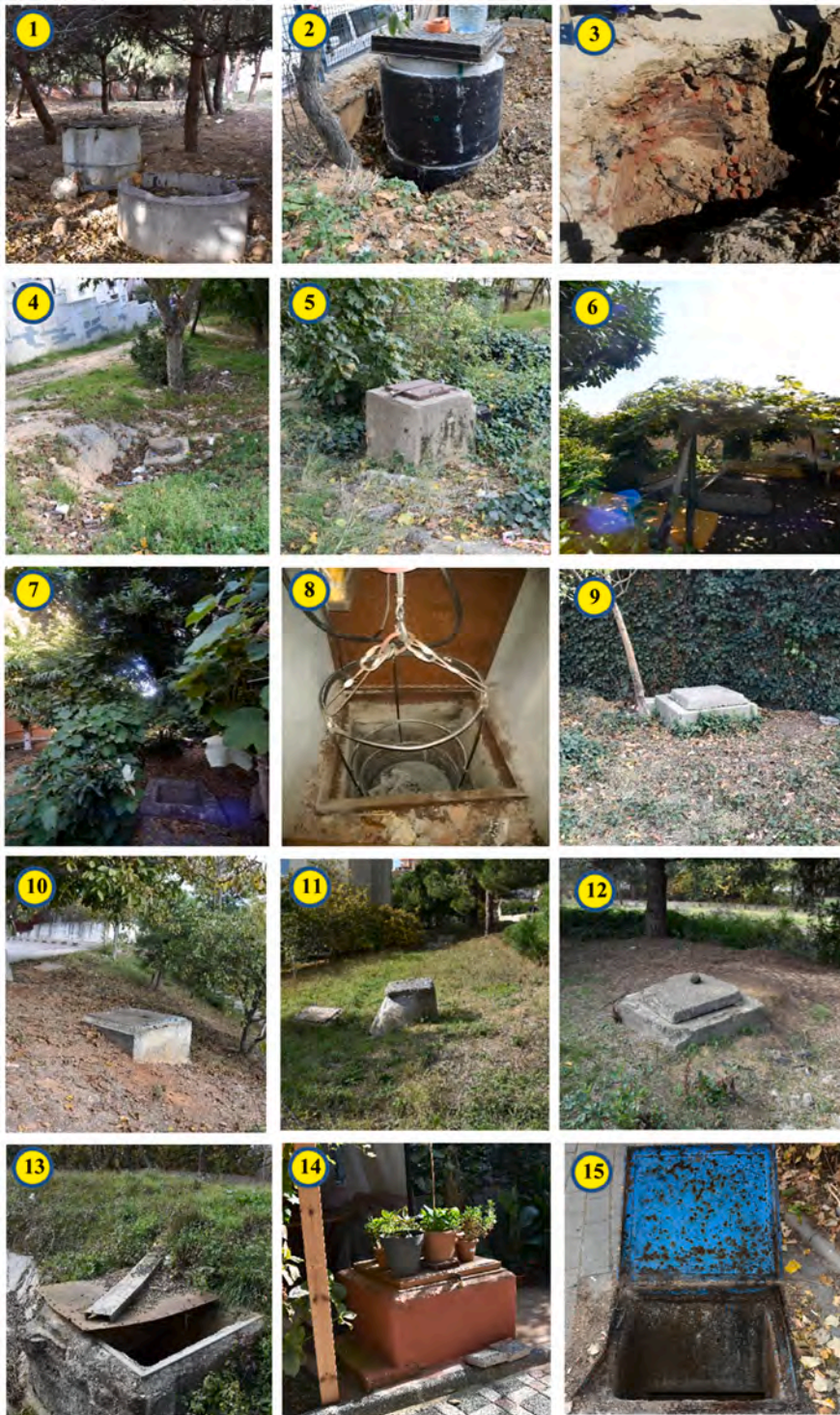
Fig. 2. . Photos of the examined shafts.
